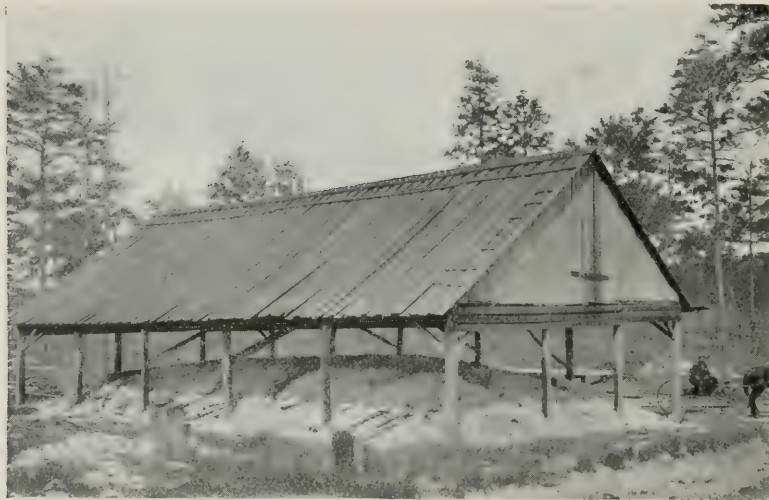
TYPICAL GRAVEL-KILN AND SHED AFTER BURNING.
