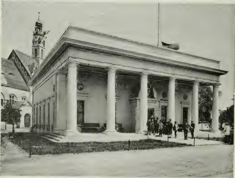
NEW SOUTH WALES BUILDING.
