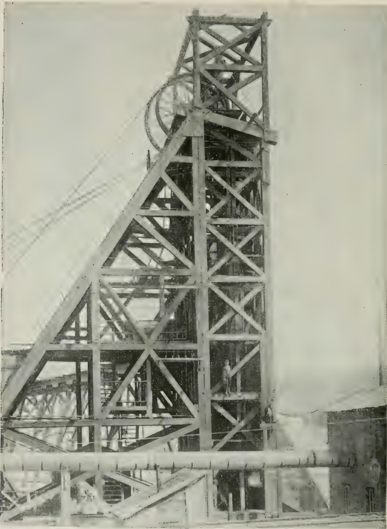
HAMILTON ORE COMPANY'S NO. 2 SHAFT HOUSE. [Looking east. Water discharging from bottom of baler.]
