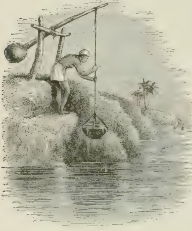
FIG. 11—EGYPTIAN SHADUF.
