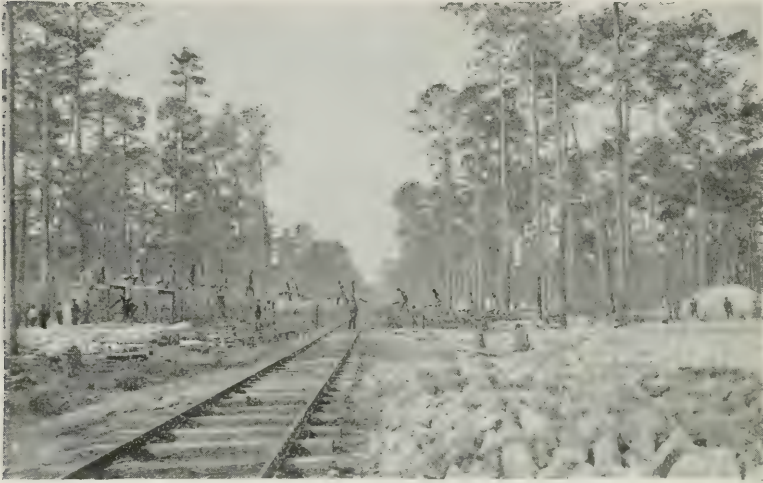
80-PER-CENT. MARION PHOSPHATE ROCK BEING SUN-DRIED, AND SCREENING FINE GRAVEL TO KILN FOR BURNING.
