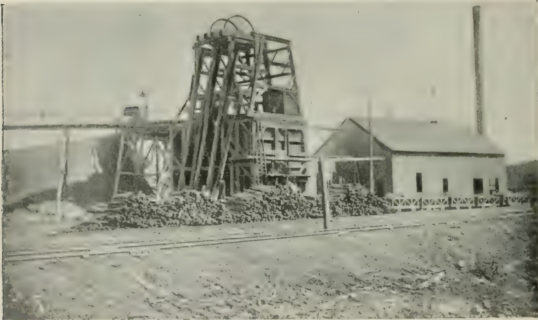
NO. 1 QUEEN SHAFT—LOOKING EAST.
