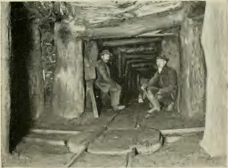
TURNTABLE IN EAST NORRIE MINE. [Timbers Showing Weight and Beginning to Crack.]
