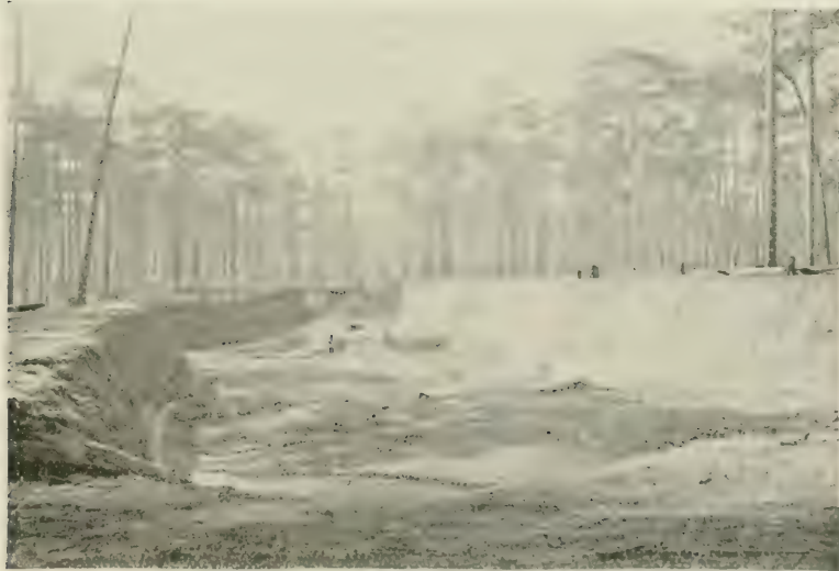
SPRATT TRACT—OVERLIE DEN REMOVED, READY FOR MINING.
