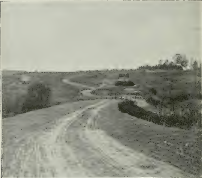
ROAD-BUILDING IN A SOUTHERN STATE—STRAIGHTENING AND GRADING.
