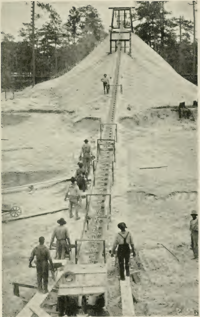
THE "GOPHER" MACHINE REMOVING OVERBURDEN OF SAND.
