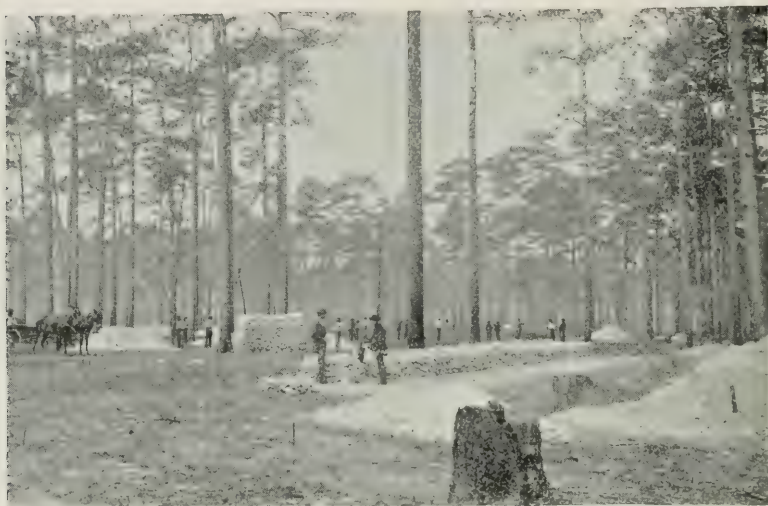
PROSPECT TRENCH AND SHAFTS AT ROCK SPRINGS TRACT, FLORIDA.
