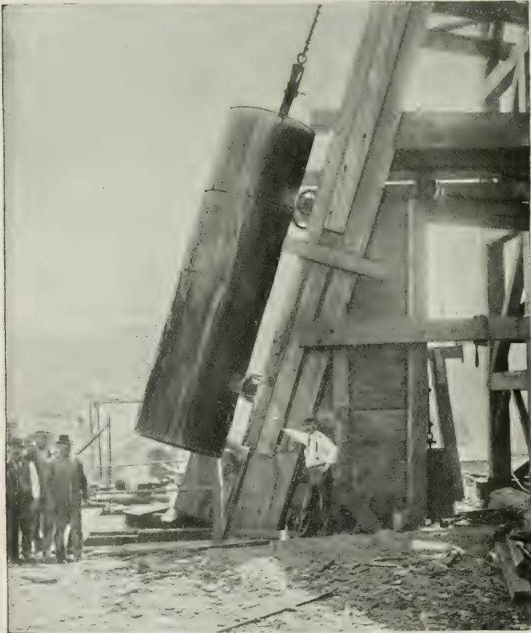
WATER DISCHARGING FROM SMALL BALER OF LUDINGTON MINE.
