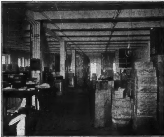
FIG. 3.—A CORNER ON THE SECOND FLOOR OF THE ELECTRIC APPLIANCE COMPANY'S NEW BUILDING.
